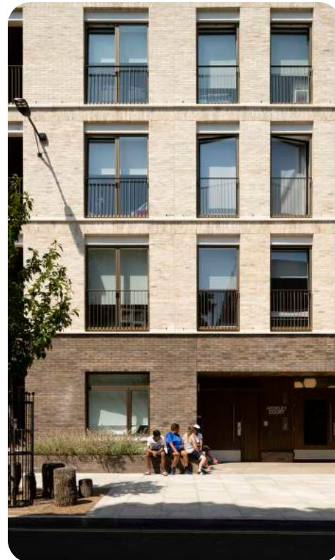
Pedestrian Entrances Precedent of Kings Crescent
