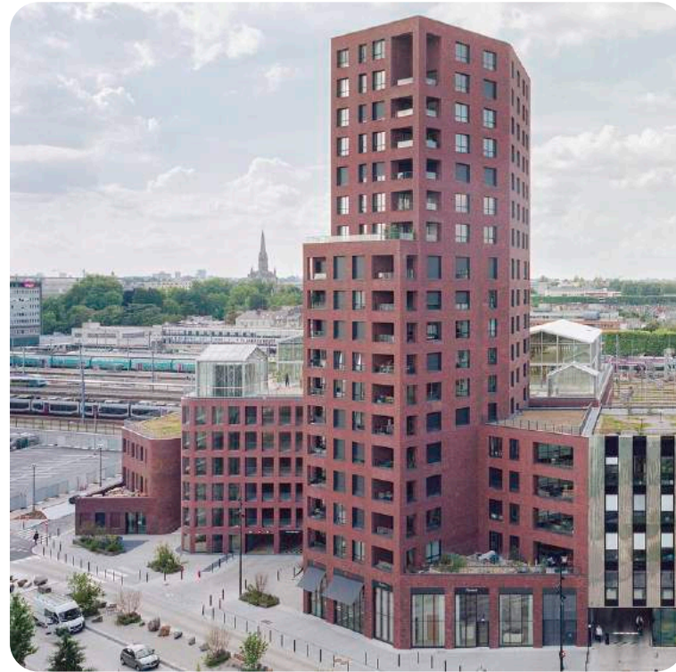
Chamfers Precedent Block 5B RAUM, France
