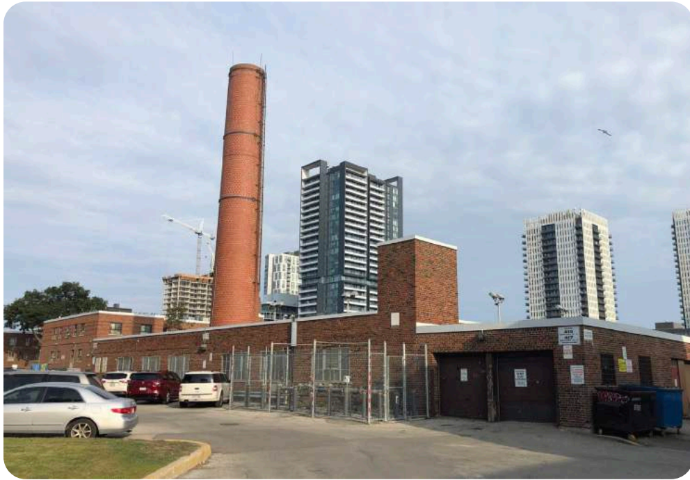
Boiler House, Regent Park
