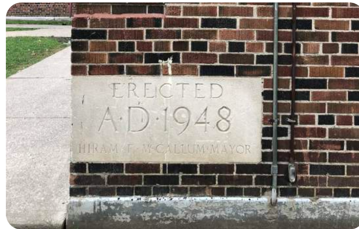
Regent Park cornerstone. Source: ERA Architects
