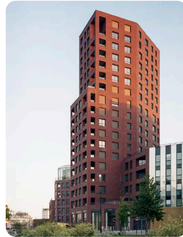
Chamfers Precedent Block 5B RAUM, France
